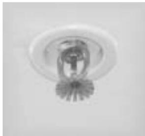
Fire sprinkler systems are based upon a series of pipes with heat activated heads that are located on or near the ceiling spaces in the roof areas of the building. At a certain temperature (well above the likely ambient temperatures for the building), the heat will cause the sprinkler head to release the water and control the spread of fire.
