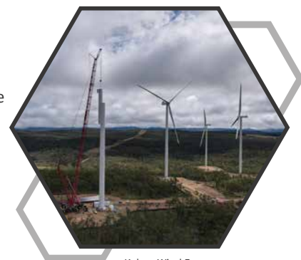
Kaban Wind Farm.
