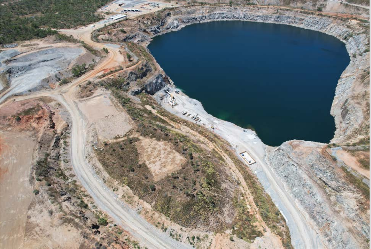
Kidston Pumped Storage Hydro Project (K2-Hydro), including the existing open-cut pit that is being repurposed.
