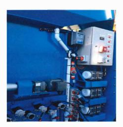
Individual Air Pumps operate in each tank, providing regulated air through the Dissolved Oxygen Metre.
