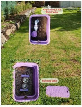
Figure 7 ABSORBS<sup>TM</sup> system showing valve boxes with sequencing, air relief and flushing valves
